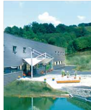
interscience R&D center and manufacturing plant
